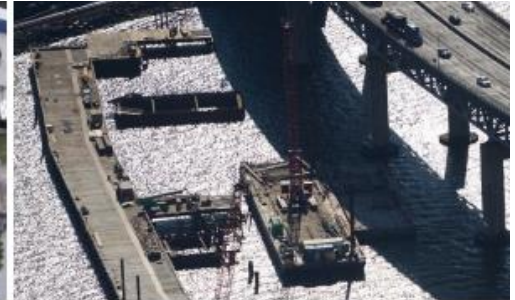
Cofferdams for New Tapan Zee Bridge, NY
