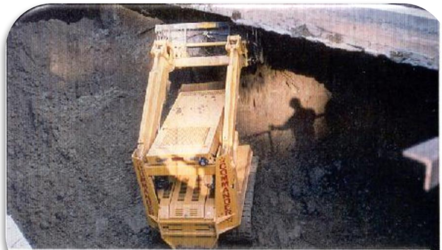
Excavating Under The Grade Level Slab
