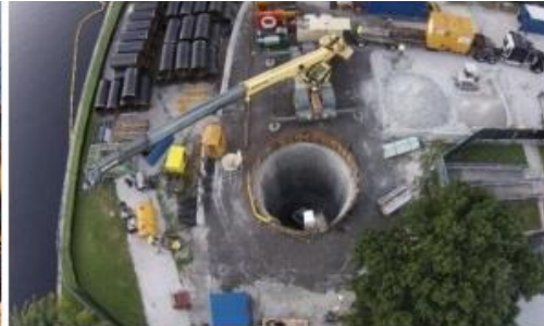
Circular wet soil mix shaft, Florida
